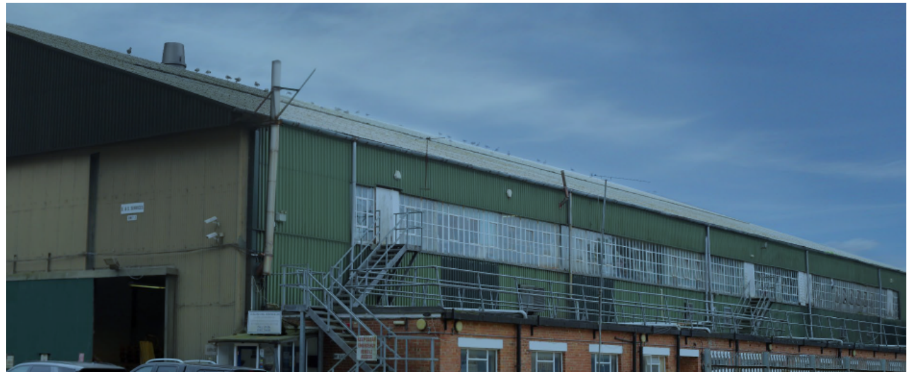
View from the West >
